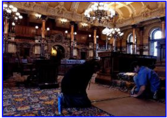
Anthony S. Bush/The Capital-Journal Derrick Willard, left, and Matt Gockel, employees of BA Designs, tape down boards to protect the new carpet in the Senate chamber at the Statehouse before heavy furniture was moved through the chamber. Click here to check for reprint availability.
